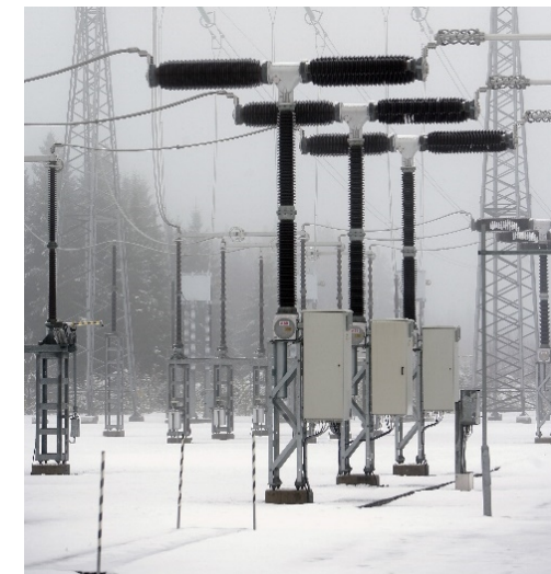
Plate 5.9 – Typical HVAC Circuit Breaker Image: ©ABB
