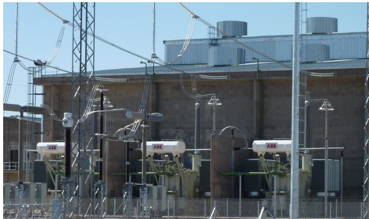
Plate 5.14 – Typical Interface transformers Image: ©ABB
