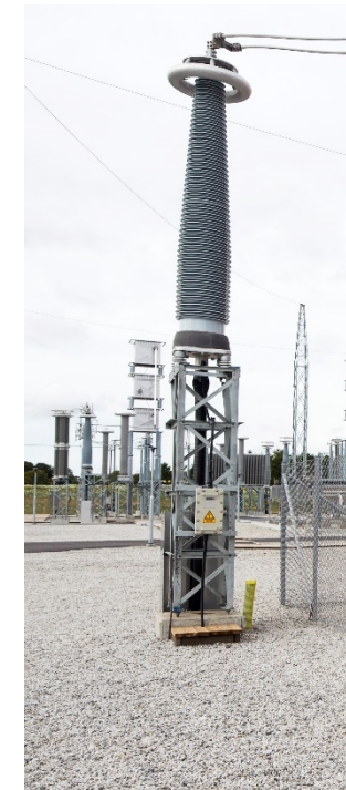
Plate 5.6 – Typical 400kV Cable Terminations Image: ©GE
