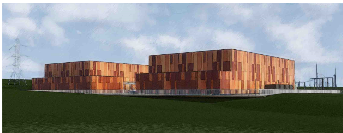
Plate 4.5 – Vertically arranged brown cladding
