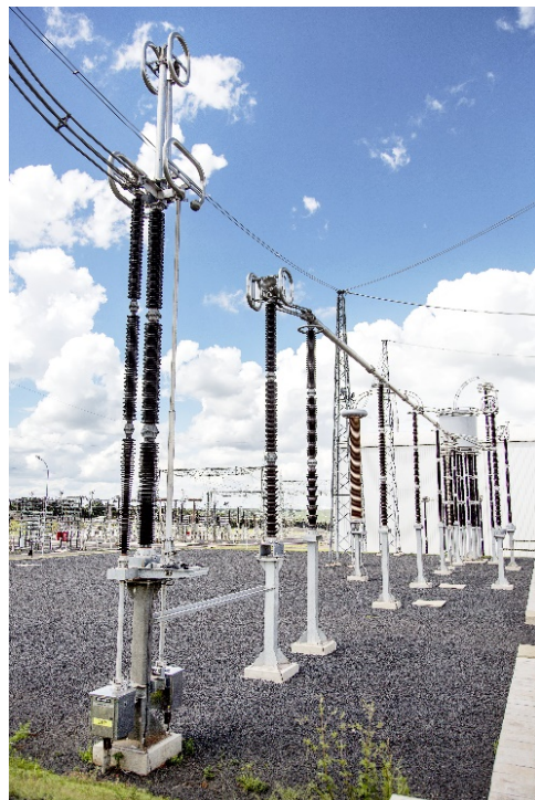
Plate 5.10 – Typical HVAC Disconnector Image: ©ABB
