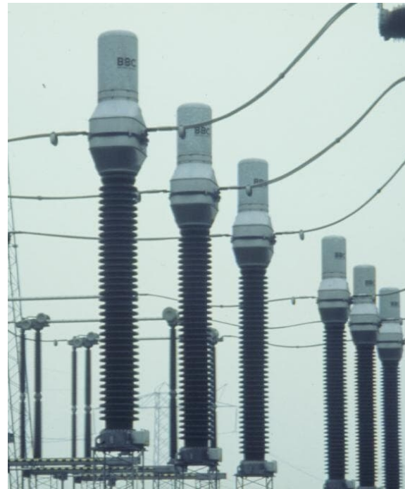
Plate 5.15 – Typical Current Transformer Image: ©ABB
